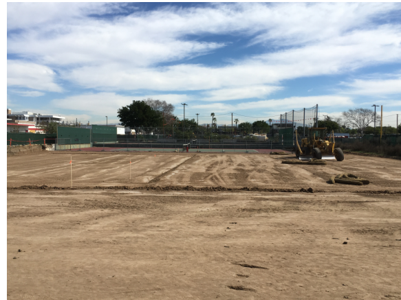
Re-compaction, fine grading and certification of new Central Plant Building pad
