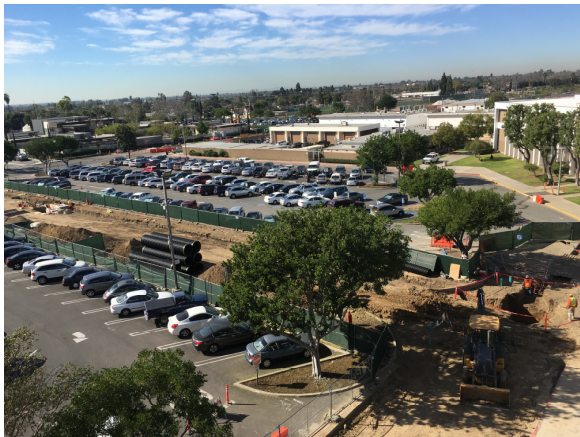
Installation of new electrical and signal conduit at Phase 1
